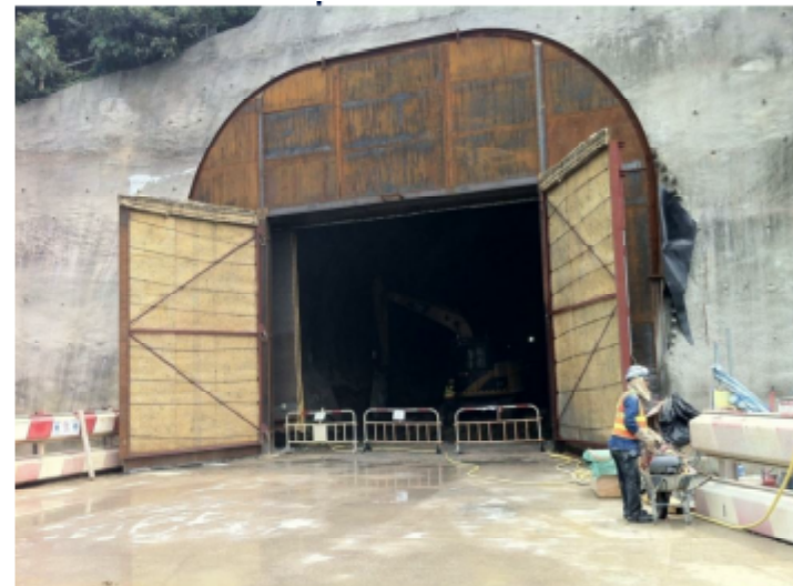
vehicular access adit (blast door)
