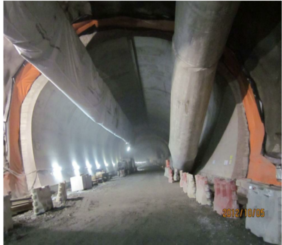
permanent lining completed with waterproofing
