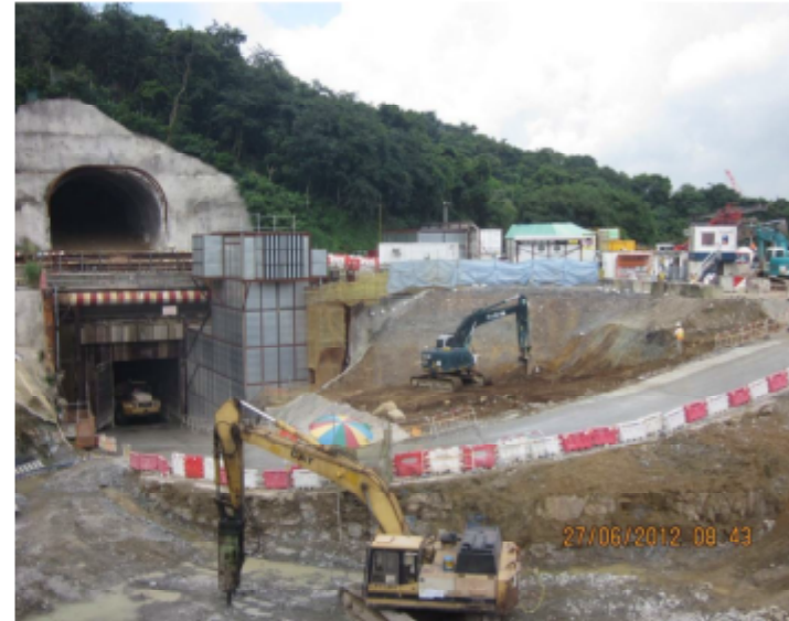
Temporary Access Ramp & Steel Platform Deck
