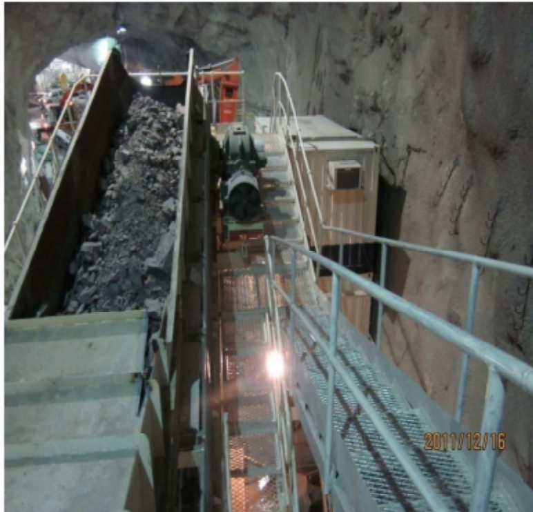
crusher and conveyor
