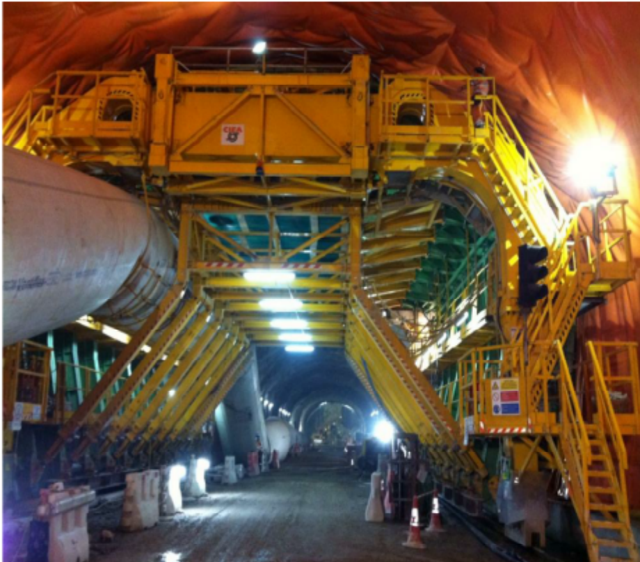
lining formwork shutter
