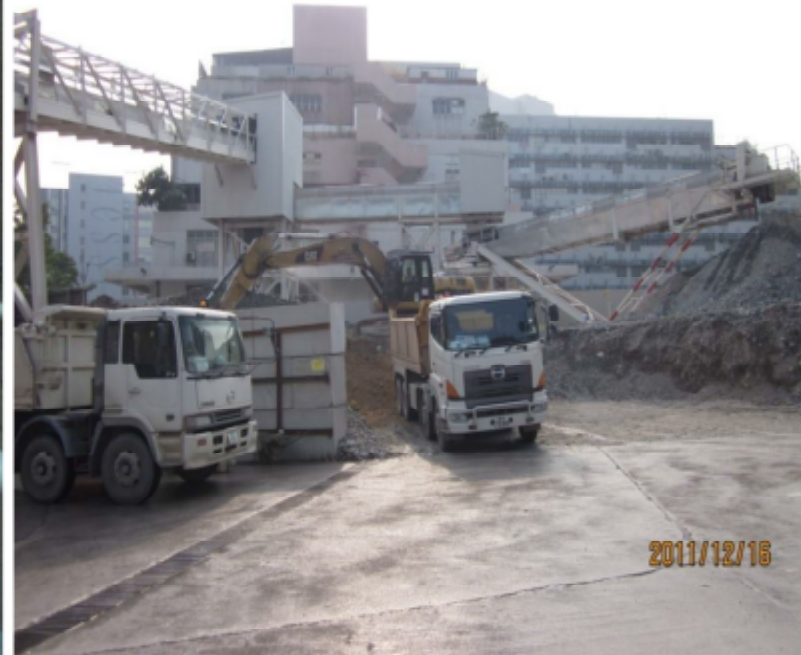
conveyor and spoil stockpile
